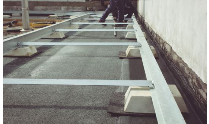
Installation of the rail track. This one has to be a freely laid track without any penetration on the roof in order not to damage the water proofing.
