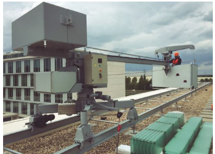
BMU FBA 1 installed in Luxembourg. Depending on the reactions that appear on the rails, these can be only supported, without fixings on the roof
