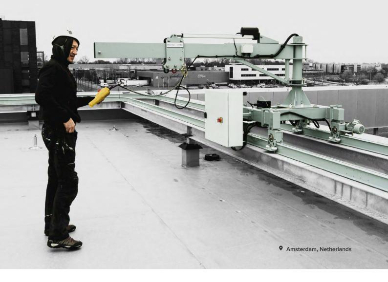
Fallprotec has designed several innovative and compact solutions for facade maintenance equipments. It is thanks to the innovations that integrate the RopeClimber person lifting hoist that a significant reduction in weight of the equipment has been achieved, among which:
